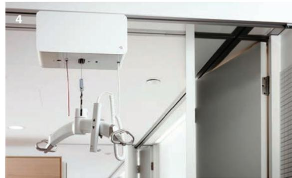
**1.** Combining Flexi's revolving/folding doors and mobile walls with a Guldmann GH3 patient lift system provides unhindered access to the entire residence. Parallel rails are built discreetly into the ceiling to function as tracks for a room covering system. This solution provides a flexible division and design of the residential space.
